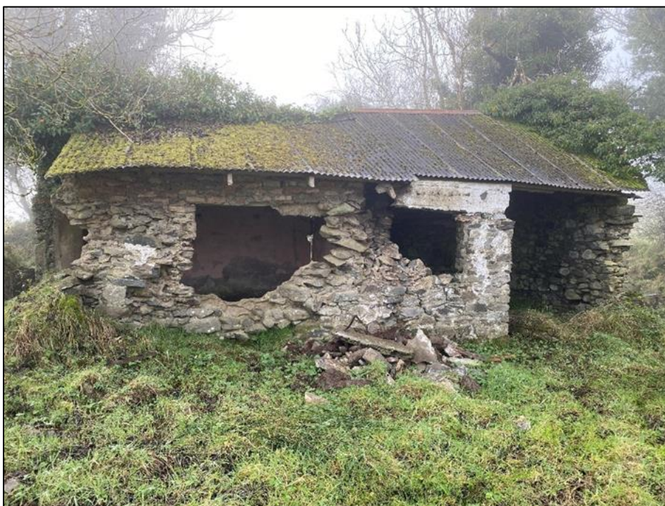
Figure 13-7: Building Eight Out-house 1 (looking west)
