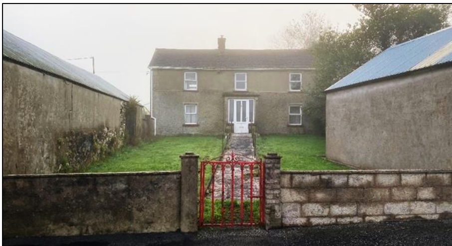
Figure 13-4: Building Six (looking southwest)
