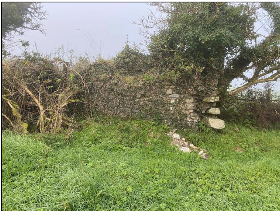
Figure 13-5: Remnants of Building Seven (looking west)
