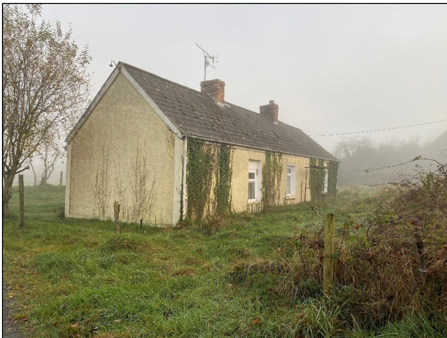
Figure 13-2: Building Three (looking west)
