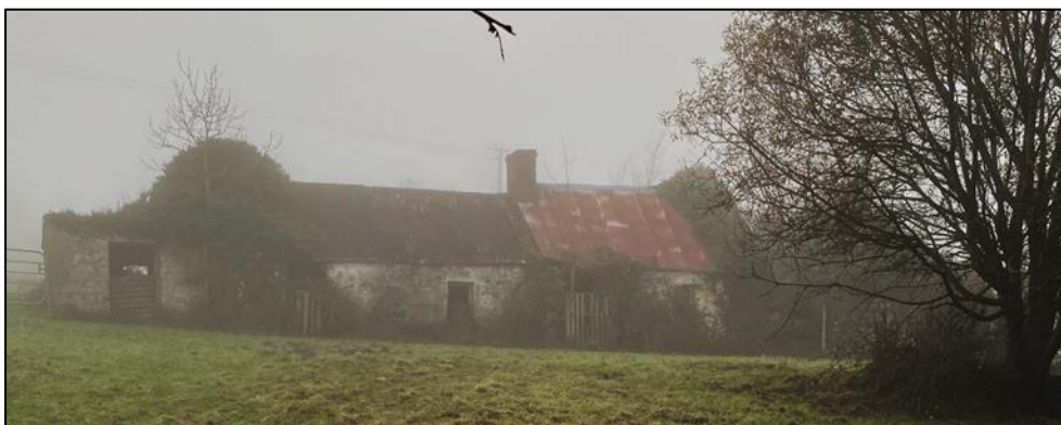
Figure 13-3: Building Five (looking southwest)
