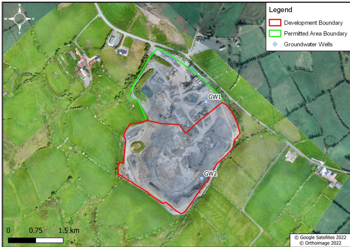
Figure 7-2: Groundwater Monitoring Wells
