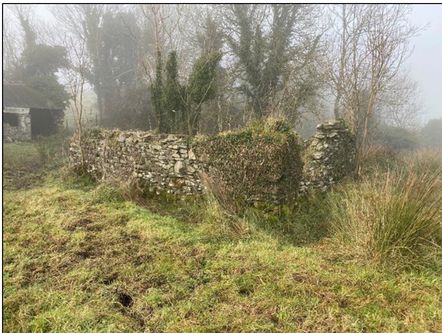
Figure 13-8: Building Eight Out-house 2 (looking west)
