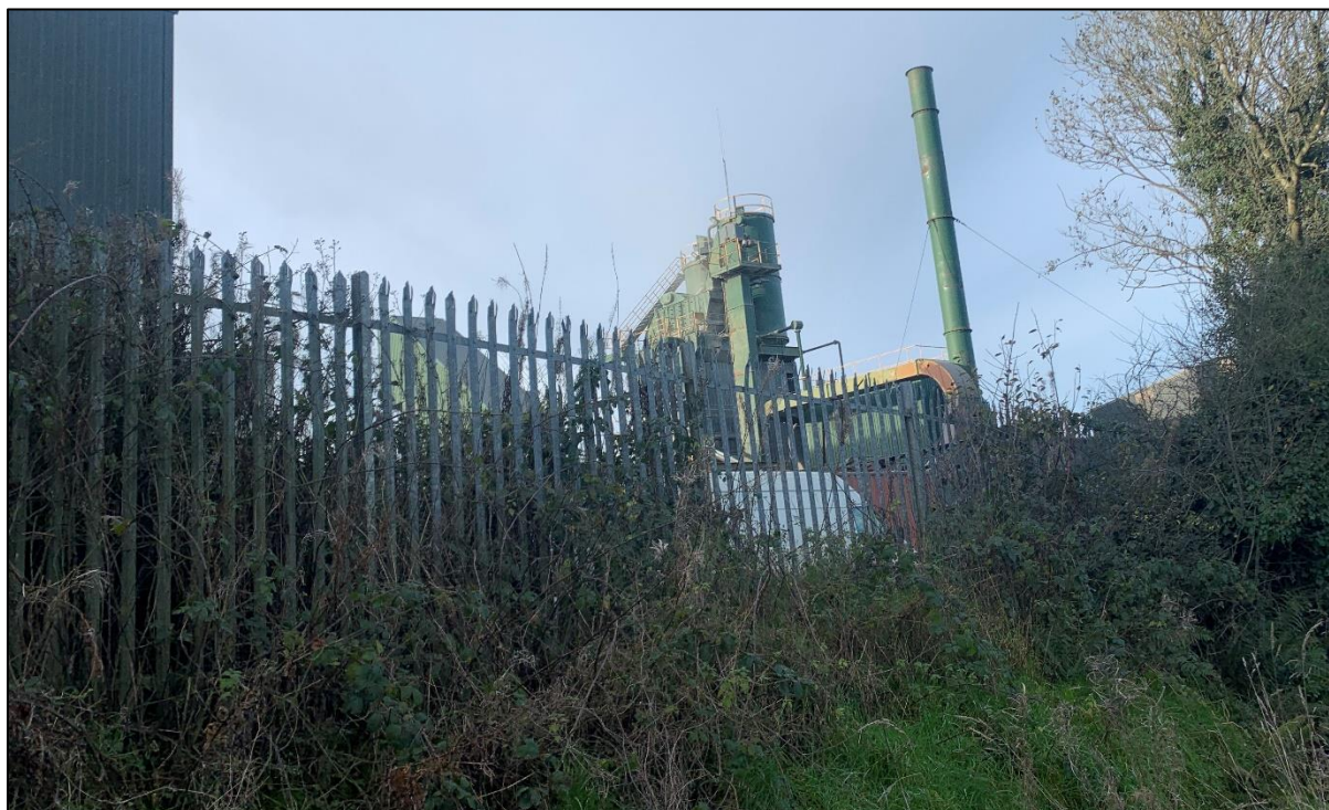
Figure 3-3: Registered Area Security Fence and Hot Macadam Plant
