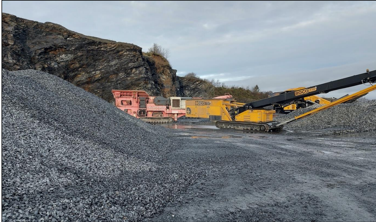
Figure 12-2: Quarry Floor, with tall quarry face to rear
